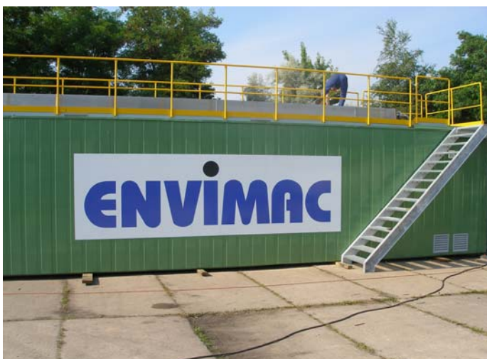
Domestic wastewater plant for 700 PE
